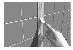
Finish the joint with caulk finishing tool. Immediately remove tape and clean up excess silicone sealant.
